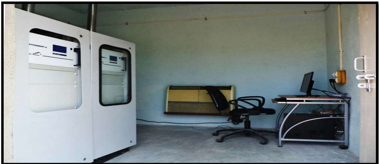
CAAQMS Station-3 installed at Mines area
