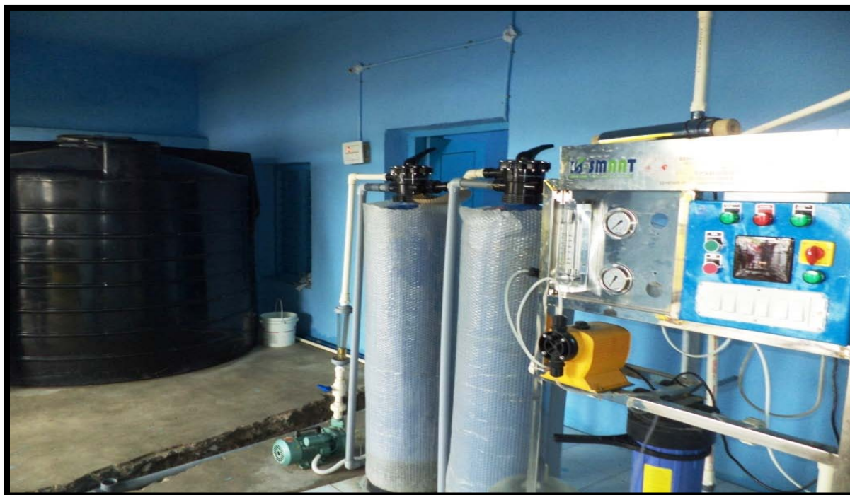
RO Water Plant Provided in Srinagar village
